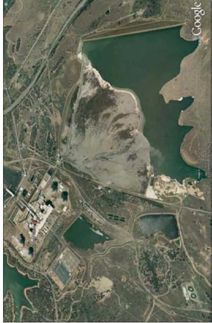
FIGURE 14: BAYSWATER POWER STATION AND ASSOCIATED ASH DAM (FOREGROUND) (SOURCE: GOOGLE EARTH)
